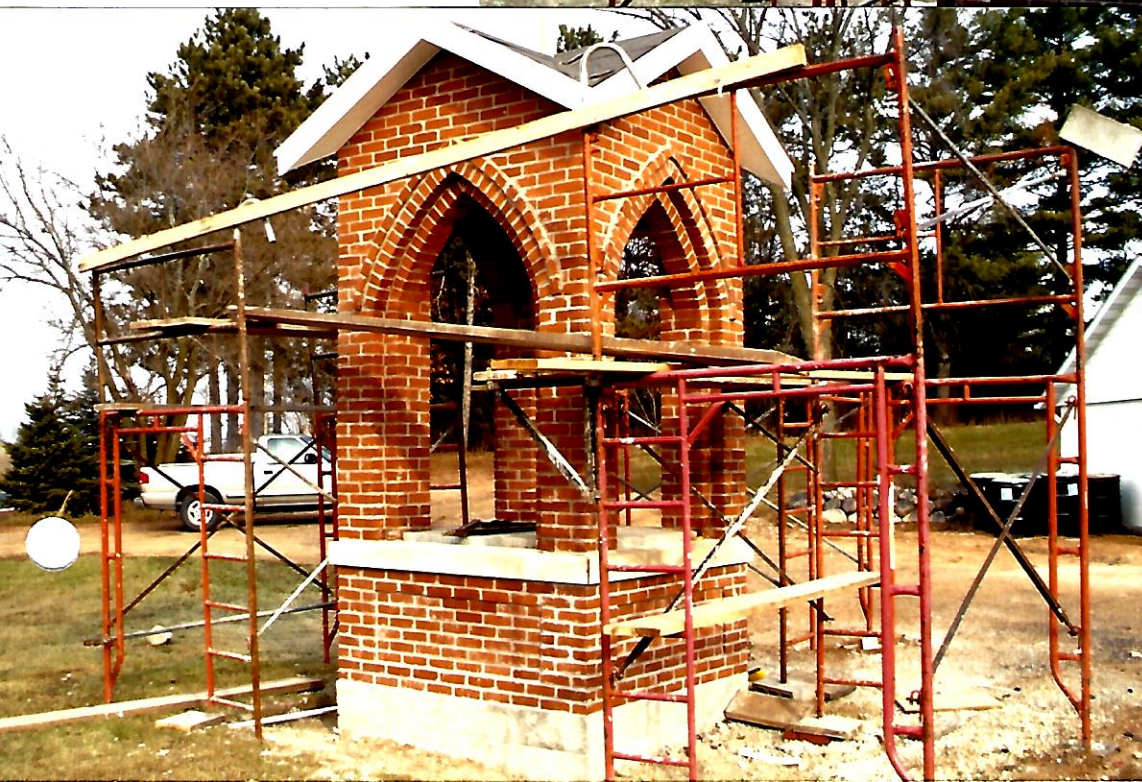
South and east side of Restored brick work
