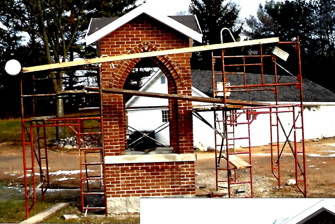
Restored brick work on south side
