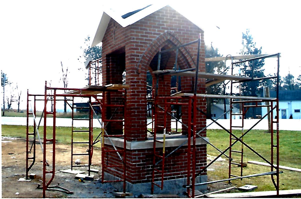
North and westside of restored brick work
